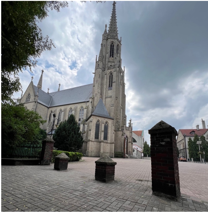
Figure 70. Concrete posts to prevent car entry while maintaining pedestrian traffic. St. Mary's Church in Katowice Source: Authors' own collections.
