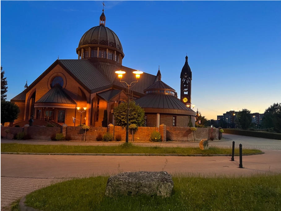
Figure 82. View of the piosts closing the access from the parking lot to the church
