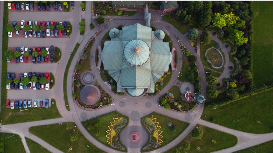
Figure 81. View of the car park at PoW
