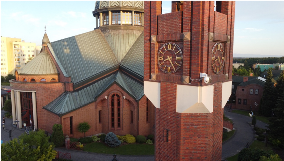
Figure 89. A rotating CCTV camera placed on the church tower for a better field of view
