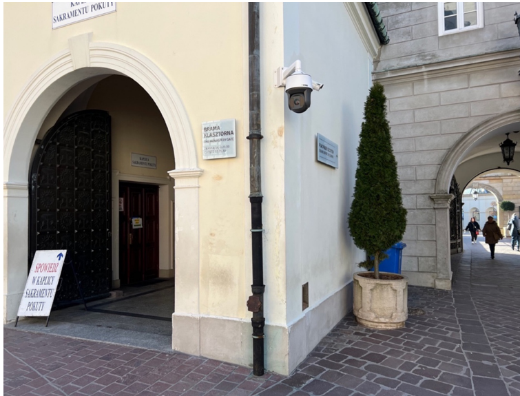
Figure 68. External rotating camera with additional stationary camera to eliminate observation blind spots. The Shrine at Jasna Góra in Częstochowa
