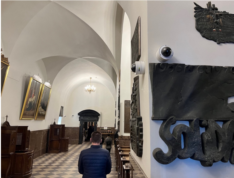
Figure 66. Cameras placed inside the PoW building in a manner that eliminates observation blind spots. The Shrine at Jasna Góra in Częstochowa
