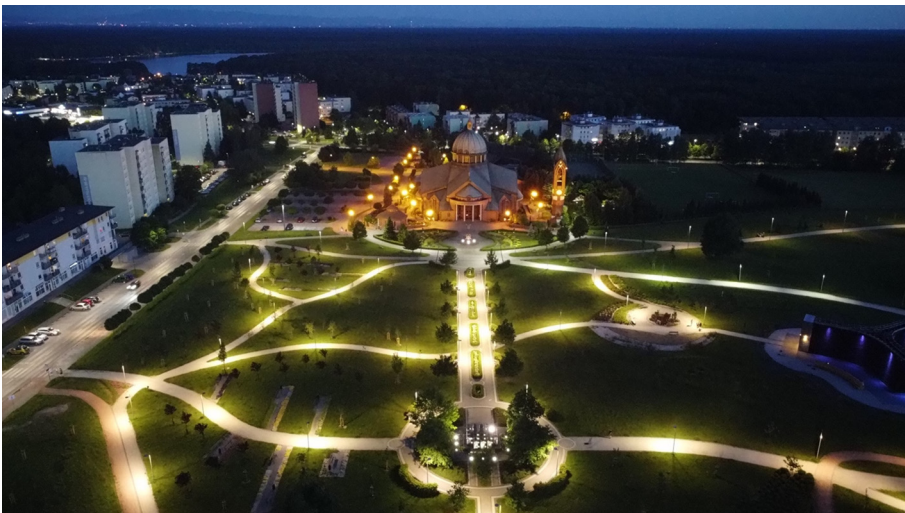
Figure 90. View of the lighting of traffic routes
