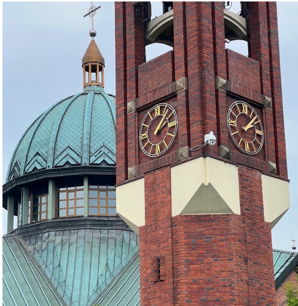
Figure 67. External rotating camera placed on the tower next to the church for more efficient observation. The Blessed Caroline Church in Tychy
