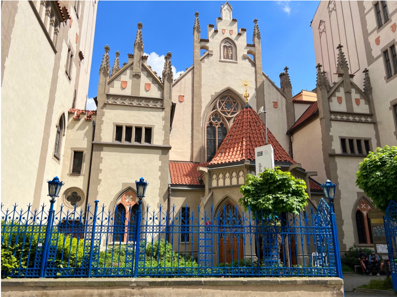
Figure 74. A metal fence with a foundation and built-in street lamps separating the synagogue building from the street in an urban compact development. The Maisel Synagogue in Prague Source: Authors' own collections.
