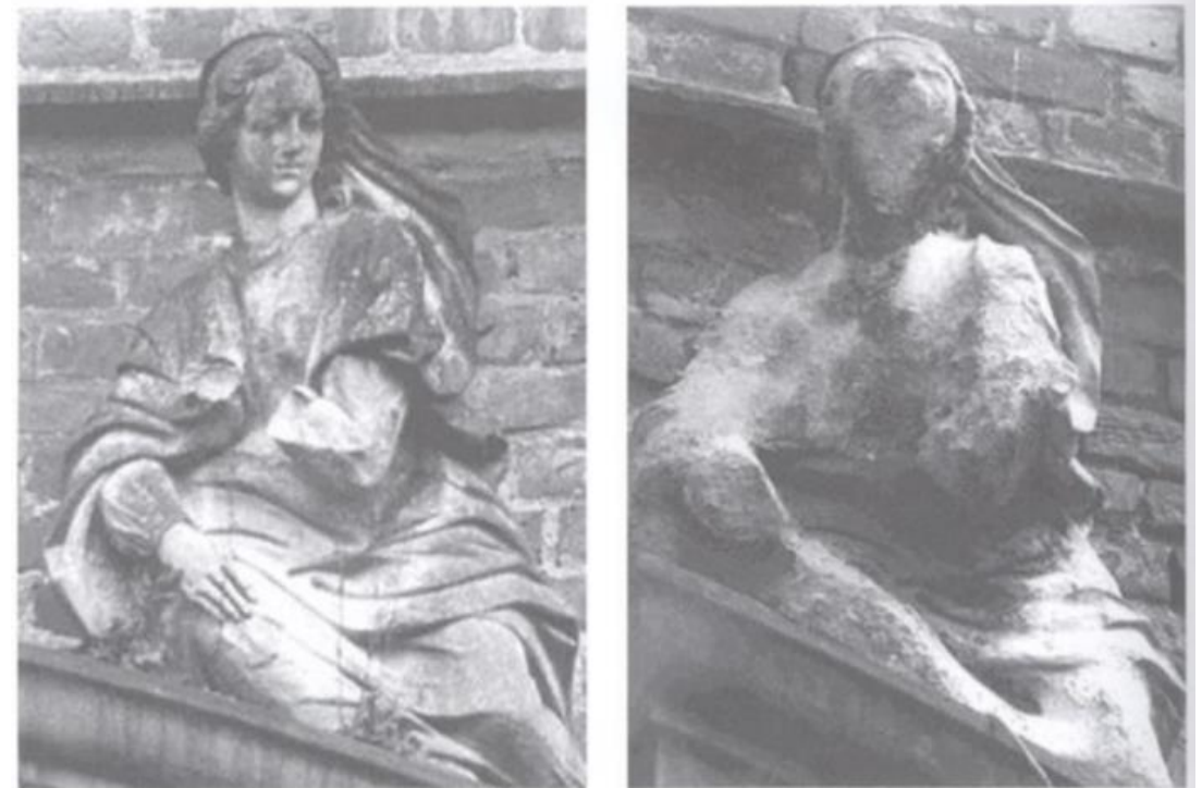
Figure 10.6. Sandstone figure over the portal of a castle, built in 1702, in Westphalia, Germany, photographed in 1908 (left) and in 1968 (right). The erosion of the figure is due to a combination of acid deposition and air pollution produced from the industrialized Ruhr region of Germany. Courtesy Herr Schmidt-Thomsen.
