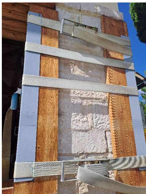
Figures 17 and 18: Temporary wall confinement system and the diagram of seismic actions acting on the building
