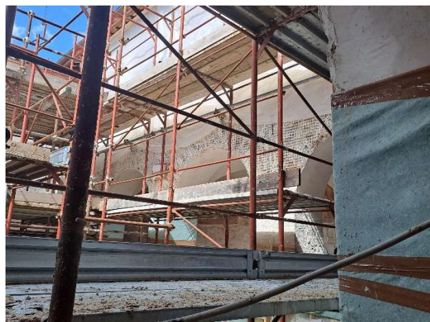
Figures 15 and 16: The current construction site and the meshes for the consolidation of wall surfaces
