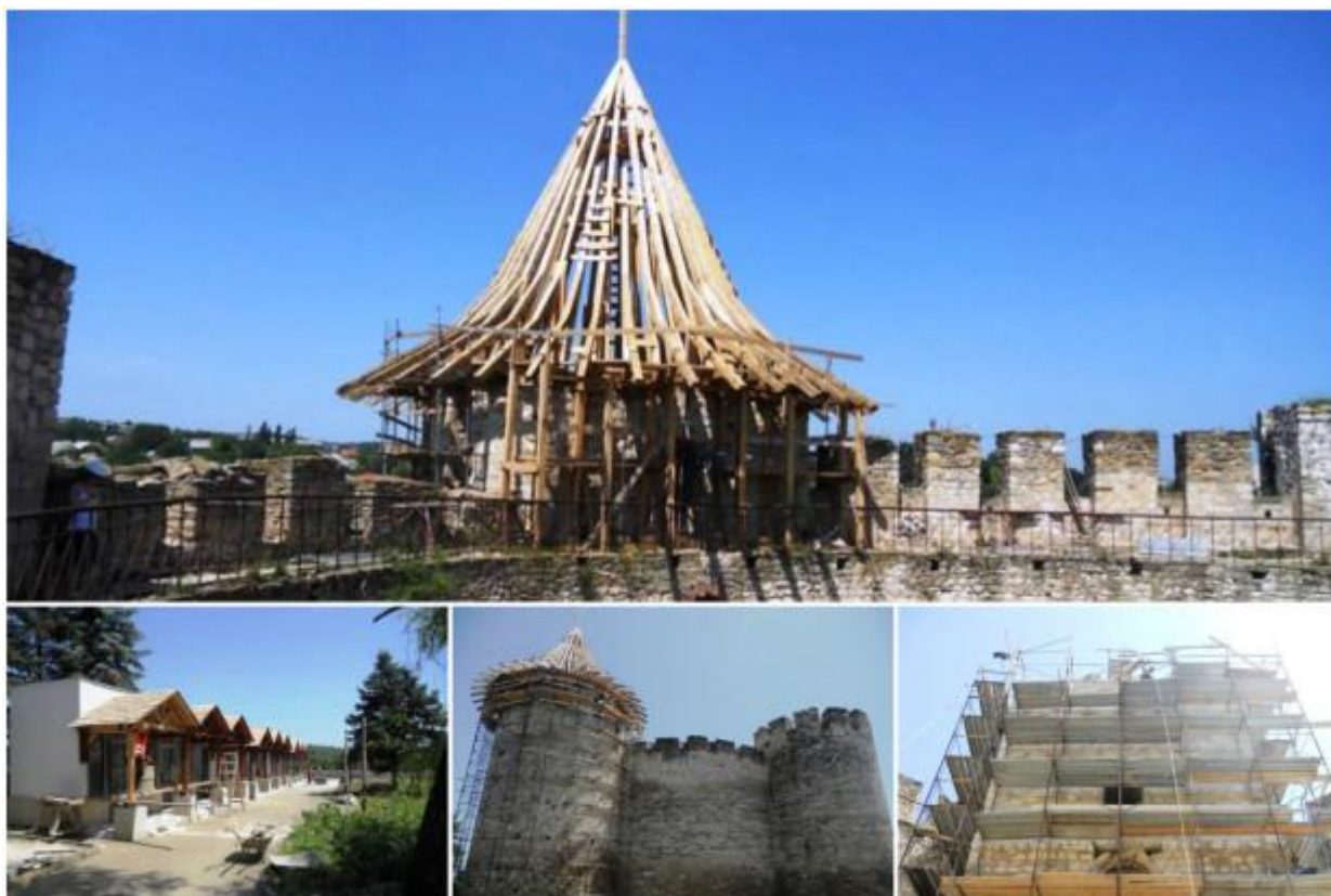
Figure 10: Restoration process of Soroca Fortress
