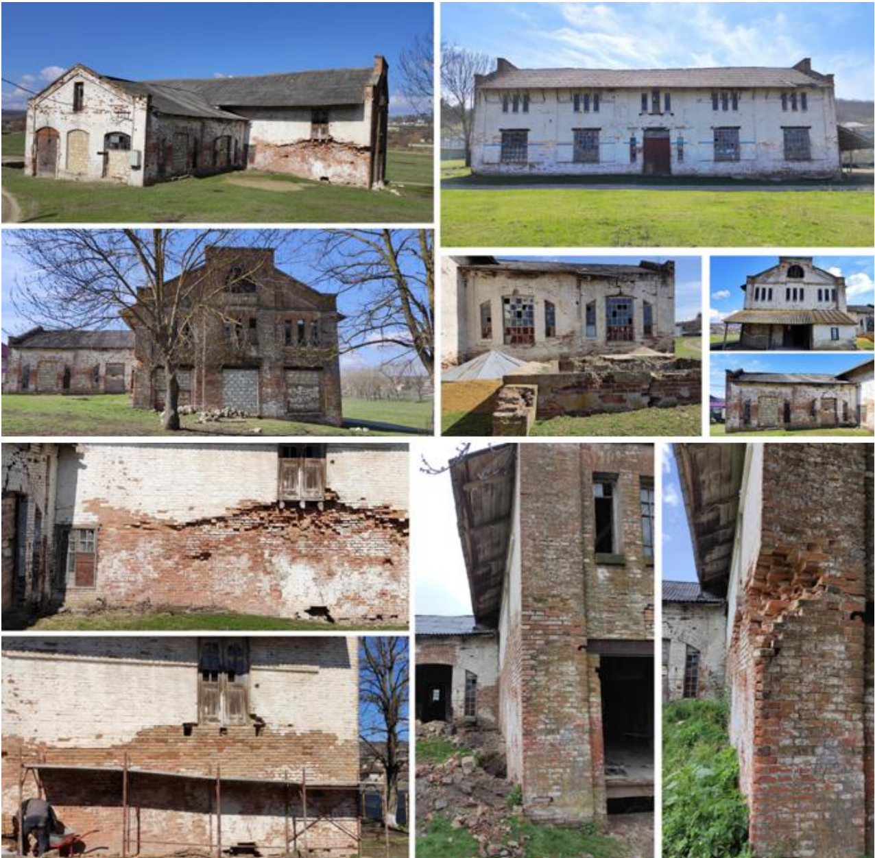
Figure 12: The building before restoration
