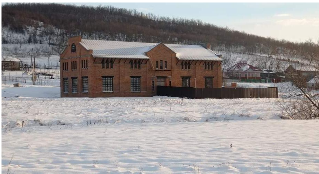
Figure 16: The end of the work. December 2023
